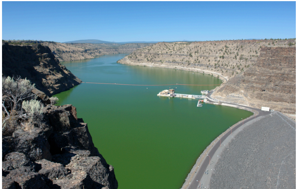
Figure 1. Surface view of the selective water withdrawal tower located in the forebay of Round Butte Dam.
